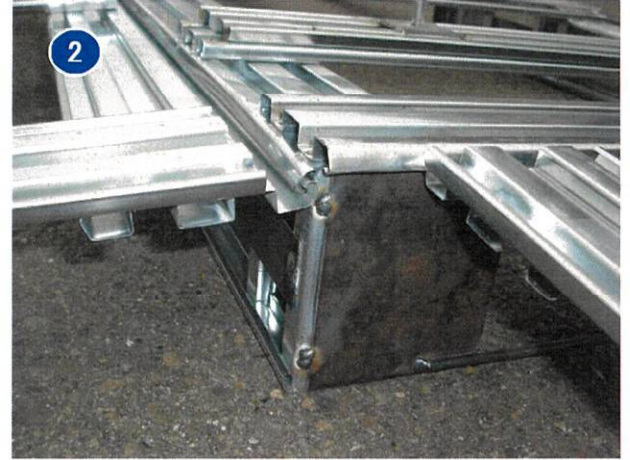
2) Setting the bottom & side boards
