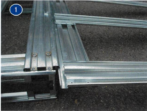
1) Setting the bottom & end boards
